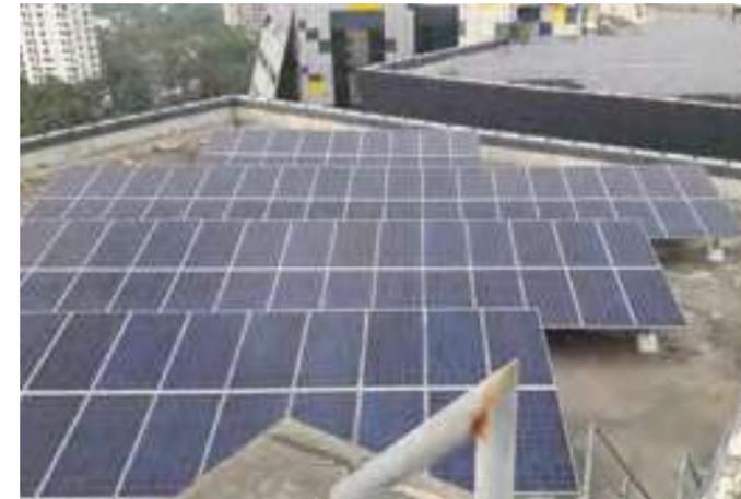
Technopark had implemented a 200kWp Roof top Grid Connected Solar Power Plant at Ganga/ Yamuna IT building Technopark Phase-III. The work was executed by KELTRON under the technical consultancy of ANERT. The project was conceived as a green initiative of Technopark and in order to partially fulfil the renewable energy purchase obligation of Technopark. The project was completed in March 2018. This plant has generated 148MWh energy till date.
